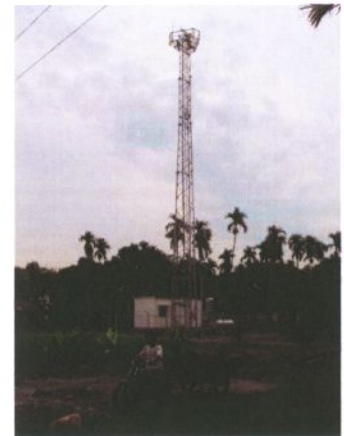
TSI Coastal Installation
